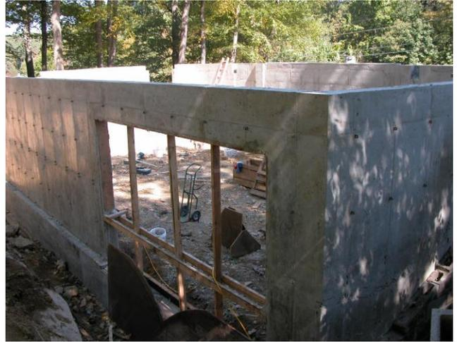
September 2004. The foundation, just uncovered from the forms. This view is of the rear (toward the reflecting pool). The doorway will lead to the public restrooms in the cellar level.
