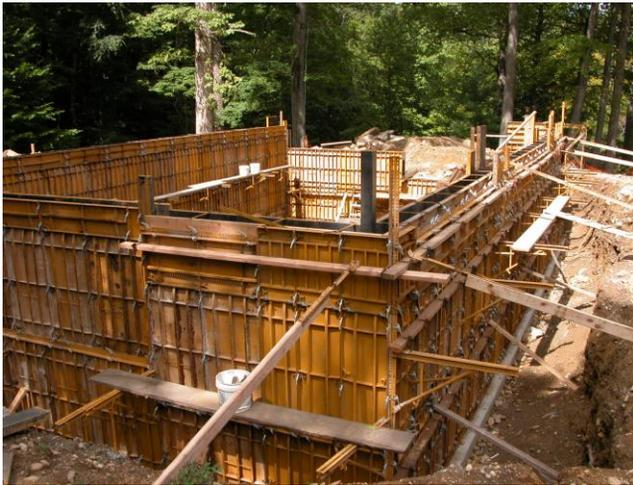
September 2004. The forms being erected. These will be filled with poured concrete. The measurements had to be exact, because the old pavilion will be re-constructed on the new foundation using the original beams.
