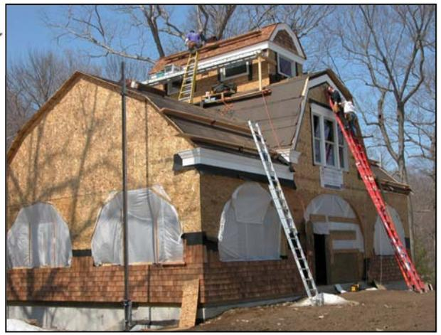
March 2005. The cedar shingle sheathing process is underway. The crew is installing trim and shingles to the pavilion. Both the roofs and the walls will be sheathed in the cedar.
