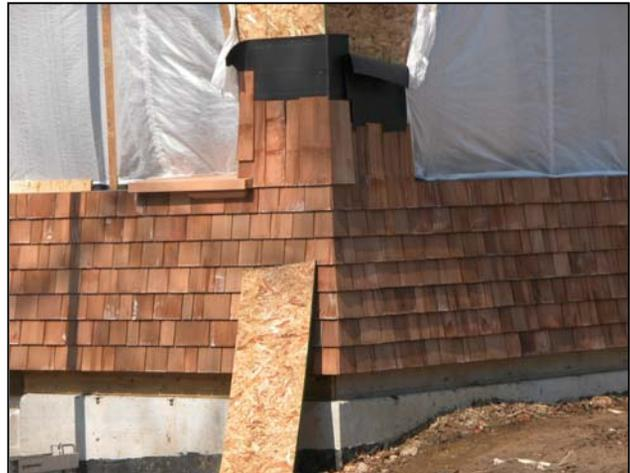
March 2005. The cedar siding has been started on all sides of the pavilion. The siding project will halt at the huge window openings, and await the installation of the custom made windows before going further up the walls.
