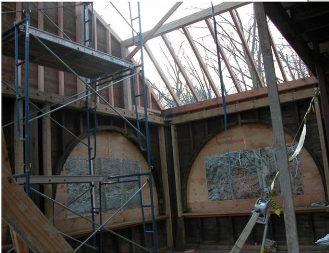
December 2004. Erecting the beams and supports in preparation for adding the second floor and the roof. New custom windows will fill the entire half-moon cut outs.
