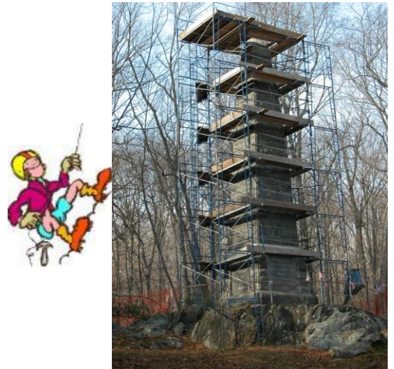
Scaffolding erected Nov. 2004
