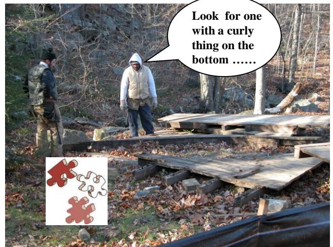
November 2004. Finding the right sections to go back into reconstruction.
