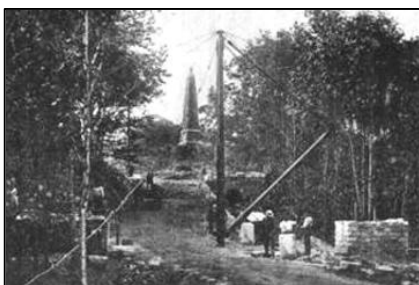
Ca. 1889, construction crews using portable crane in constructing block house at entrance.
