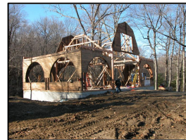
Nov - New center going up
